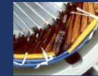
Failures in motors
