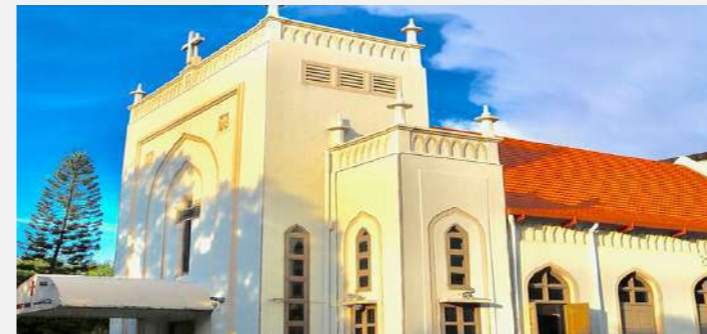
Parish of Christ Church - M&E works & Fire Protection
