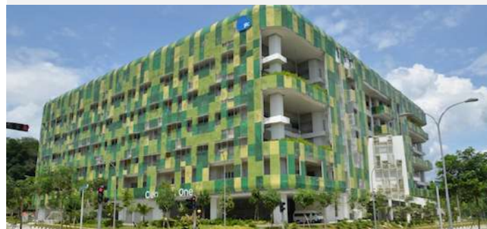
Clean tech One –Mechanical & Elect Works
