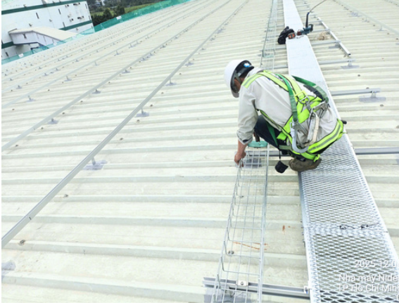
Installing DC Cable Trays
