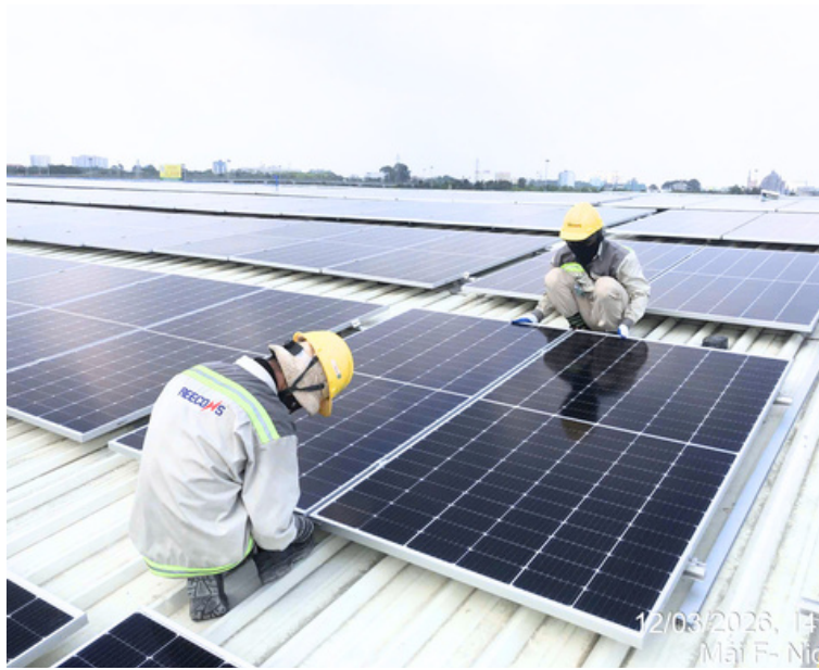
Installing PV Panels
