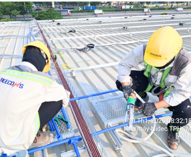
Installing Cleaning Water System
