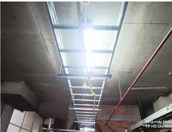
Executing AC Tray Installation
