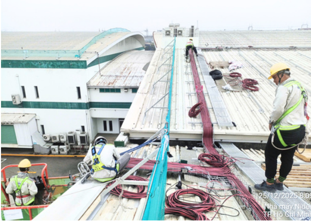
Executing DC Cable Pulling
