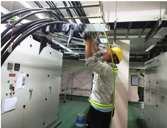
Installing AC Cabinets
