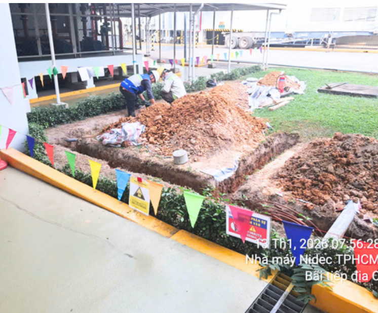
Inverter Housing Execution
