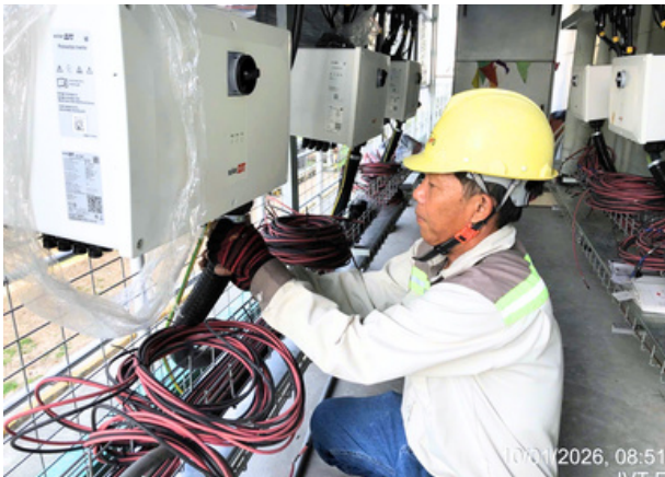
Executing IVT Installation
