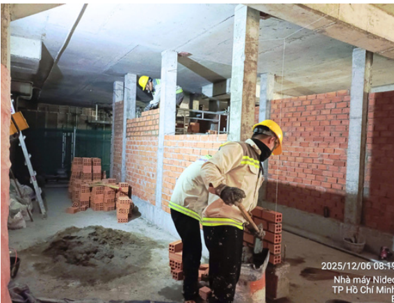
Executing IVT House Framing
