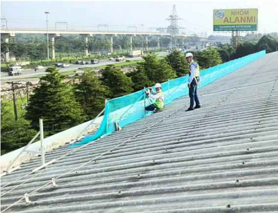
Installing Rail Frame
