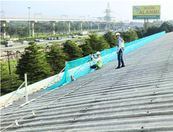
Installing Rail Frame
