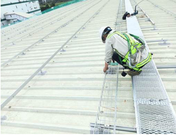
Installing DC Cable Trays
