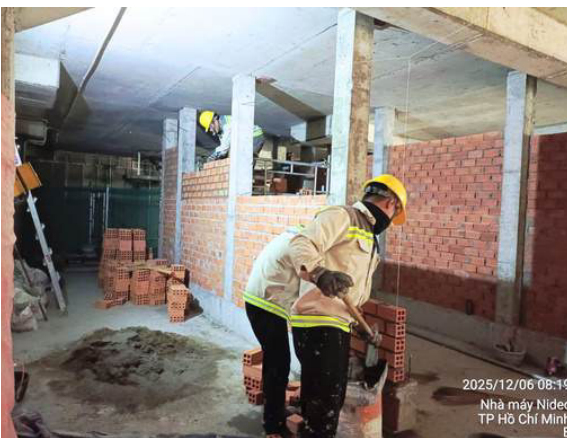
Executing IVT House Framing
