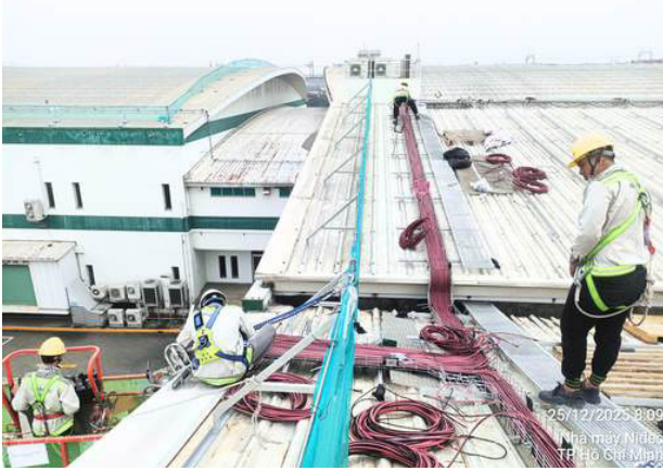
Executing DC Cable Pulling
