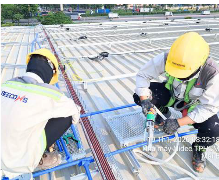
Installing Cleaning Water System
