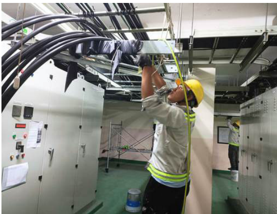
Installing AC Cabinets
