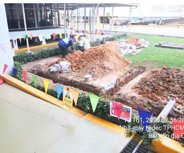
Inverter Housing Execution
