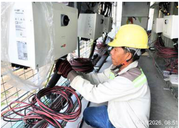
Executing IVT Installation
