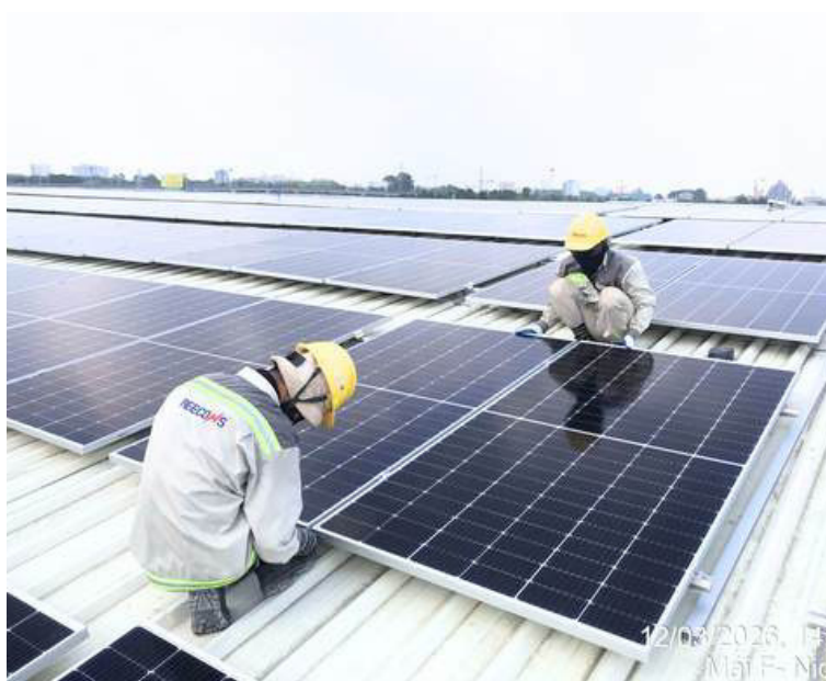
Installing PV Panels
