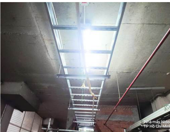
Executing AC Tray Installation
