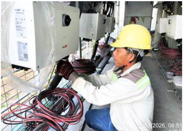
Executing IVT Installation
