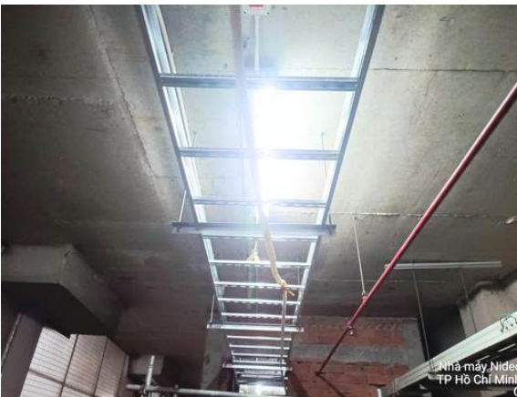
Executing AC Tray Installation
