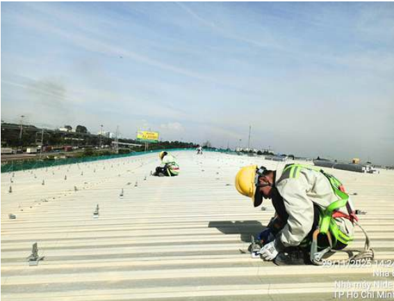
Installing Walkways
