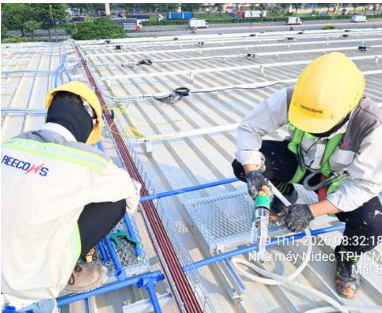
Installing Cleaning Water System
