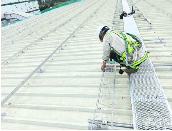
Installing DC Cable Trays
