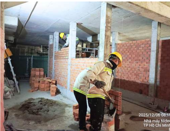
Executing IVT House Framing
