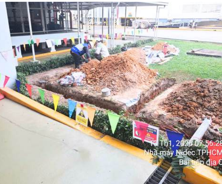
Inverter Housing Execution
