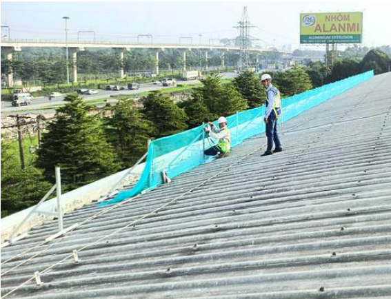
Installing Rail Frame
