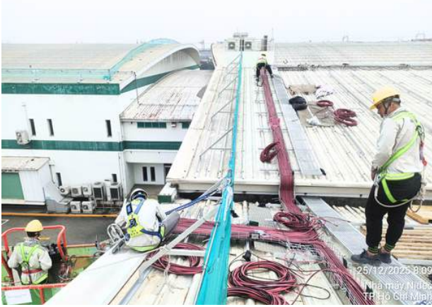
Executing DC Cable Pulling
