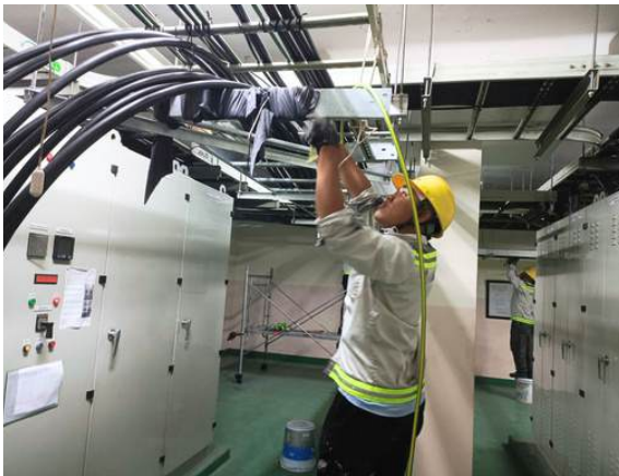
Installing AC Cabinets
