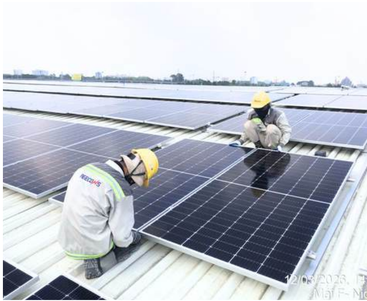
Installing PV Panels
